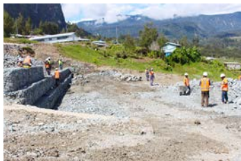
Earthworks for the construction of a 4 in 1 classroom.
