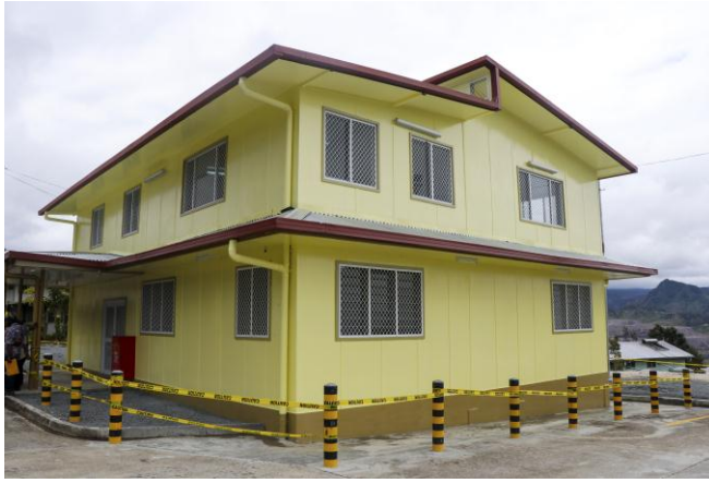
The new Paiam hospital administration building.
