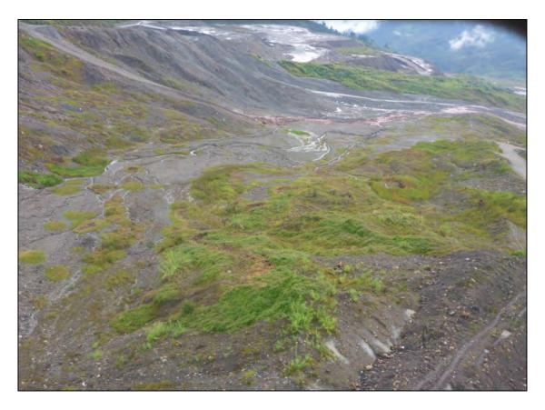
Figure 4-17 Anawe looking downstream from tip-head showing eroded and concave surface profile
