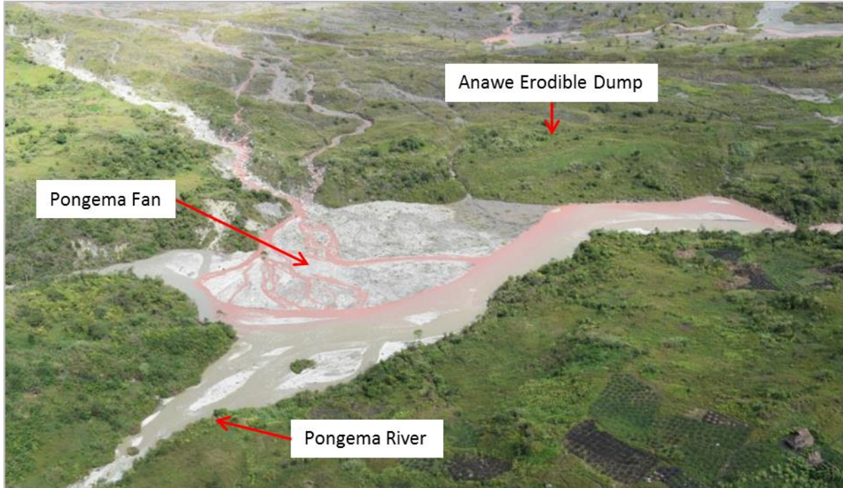
Figure 4-17 Pongema River Fan showing tailings discharge
