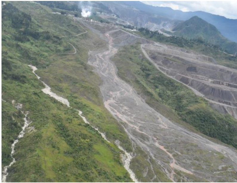
Figure 4-17 Upper Tract of Anawe Dump showing eroded surface
