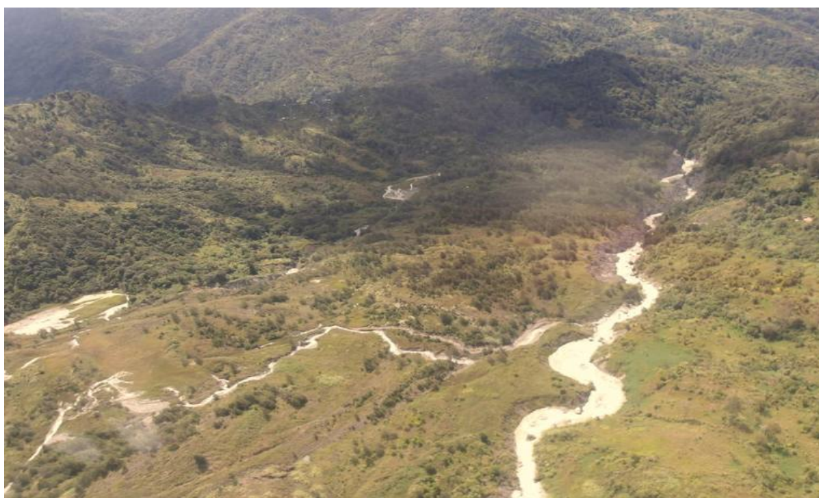
Figure 4-18 Anawe erodible dump toe
