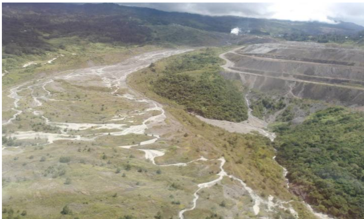
Figure 4-17 Upper Tract of Anawe Dump showing eroded surface and ‘upthrust’ zone with vegetation cover
