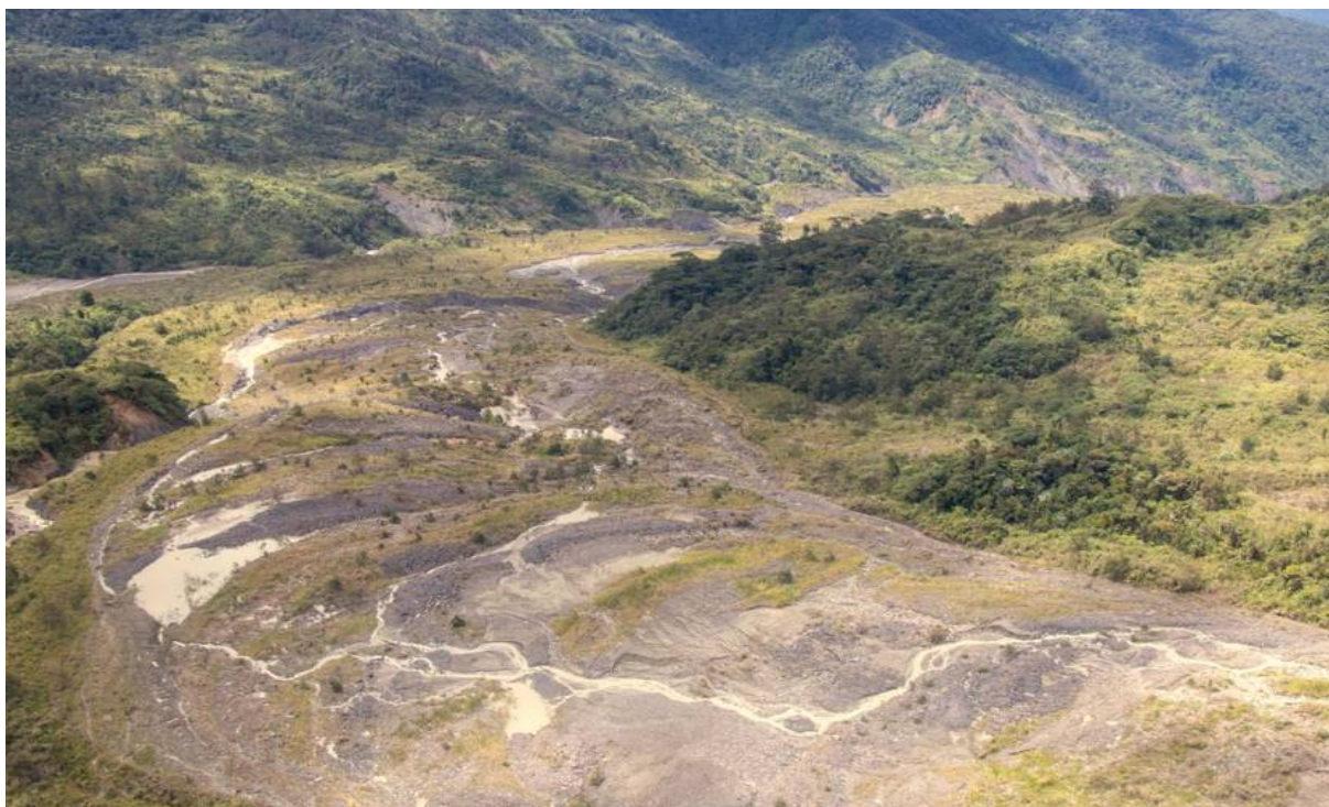
Figure 4-20 Dumped material 'rafting' downslope (view downstream from Aiyoko Ridge area)
