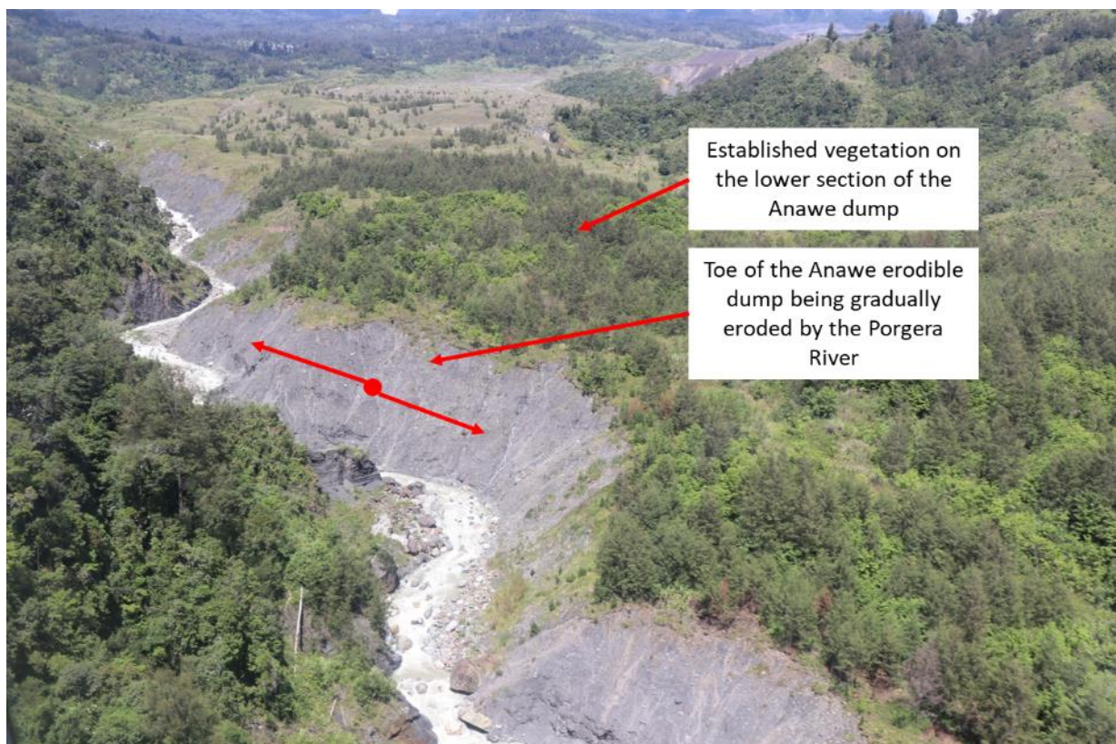
Figure 4-10 Anawe erodible dump toe intersecting the Porgera river – looking upstream towards the tip head August 2022
