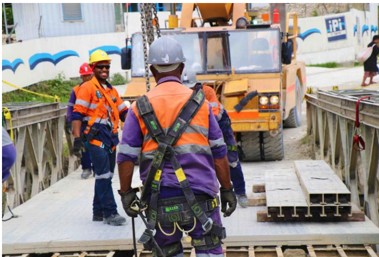
The PJV Community Projects team working on the Aipulungu bridge.
