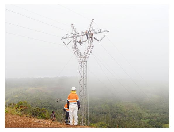
PJV Linesmen working on a new 25 metre transmission tower. Similar towers and transmission lines have been affected by vandalism.
